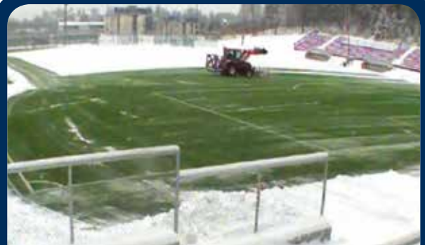
Snow is removed mechanically while the pitch is preheated. The remaining snow will melt and infill will be soft.
